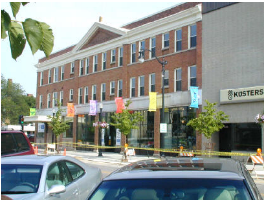
The exterior renovation brought back the buildings original character.
